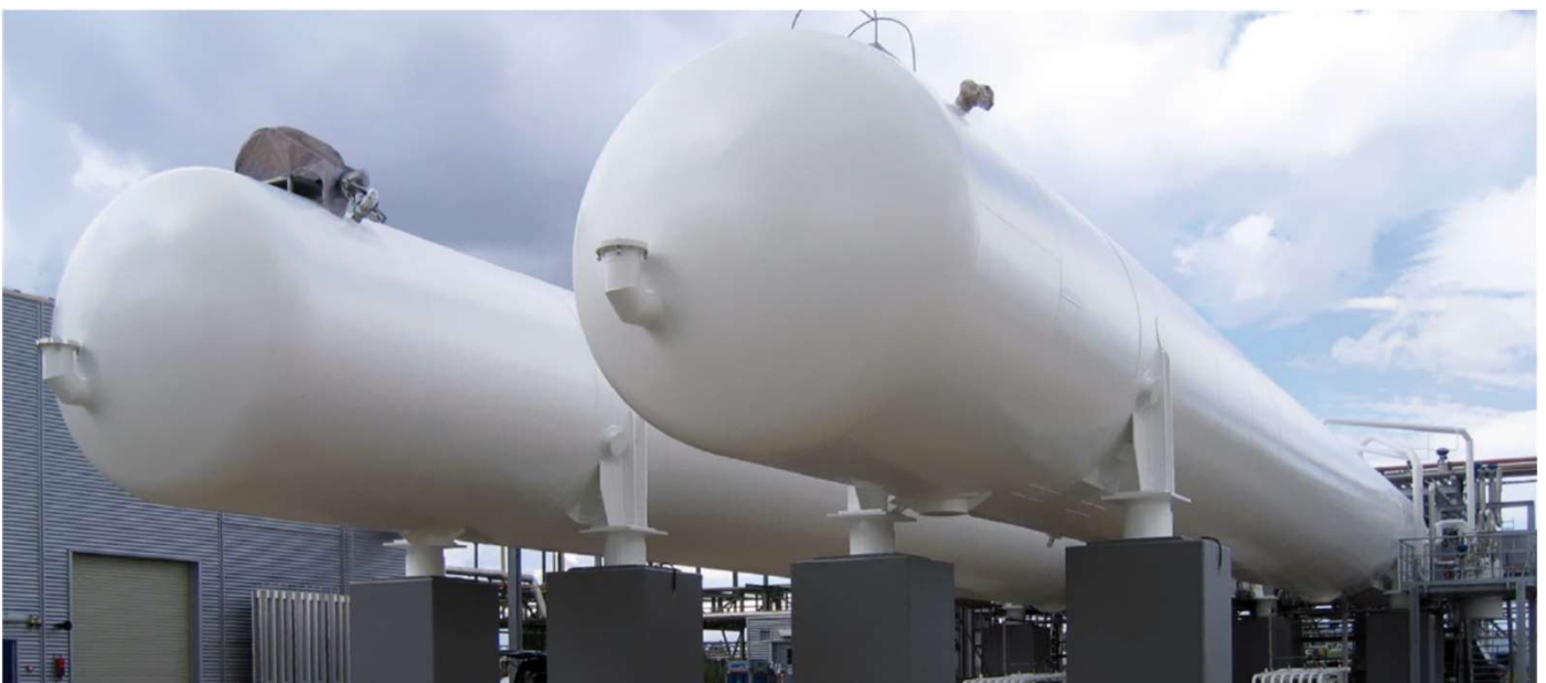
Figure 5.6: Cylindrical LH 2 tanks at the hydrogen liquefier in Leuna, Germany. Source: Linde
