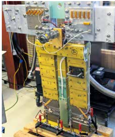
Fig. 6: Construction of the pressure-tight bushing including two 20 kA current feeds
